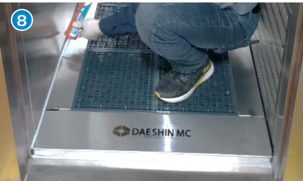
Put silicon at the edge of mat.
