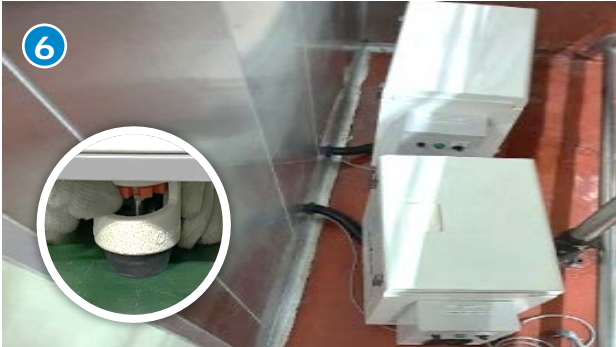
Place Dust Collector at the outside of Air Shower. Fix the wheels.
